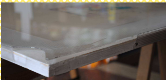
Details of the missing pieces and the biological spots of the screen
